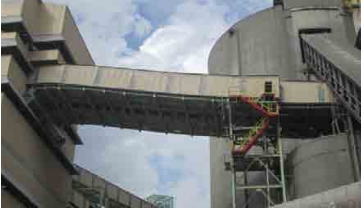
Clinker and Cement Additives Transport System Clinker and Cement Additives Transport System
