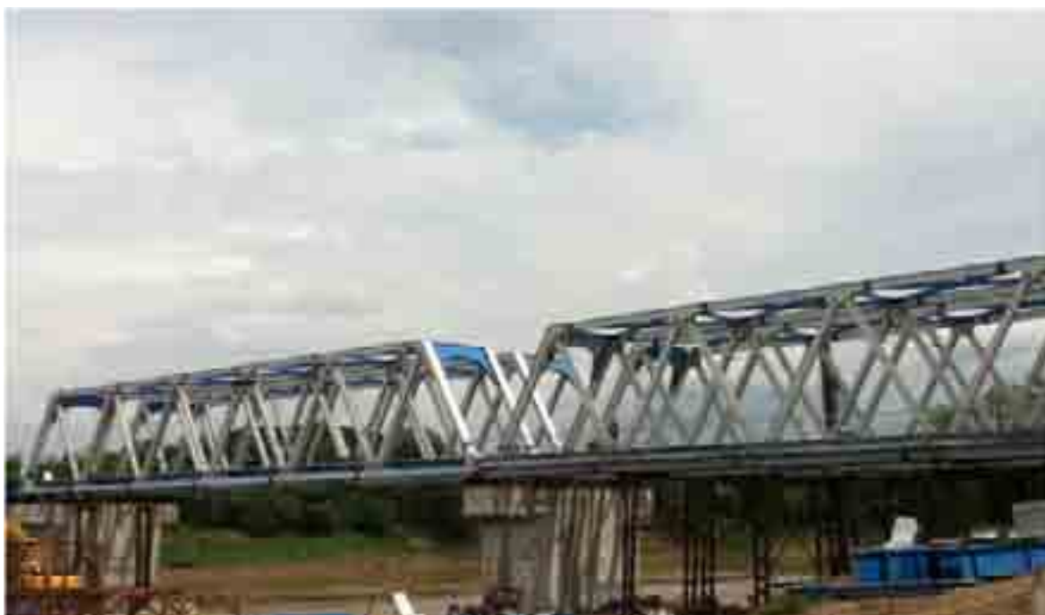
Jembatan Kereta Api Railway Bridge
