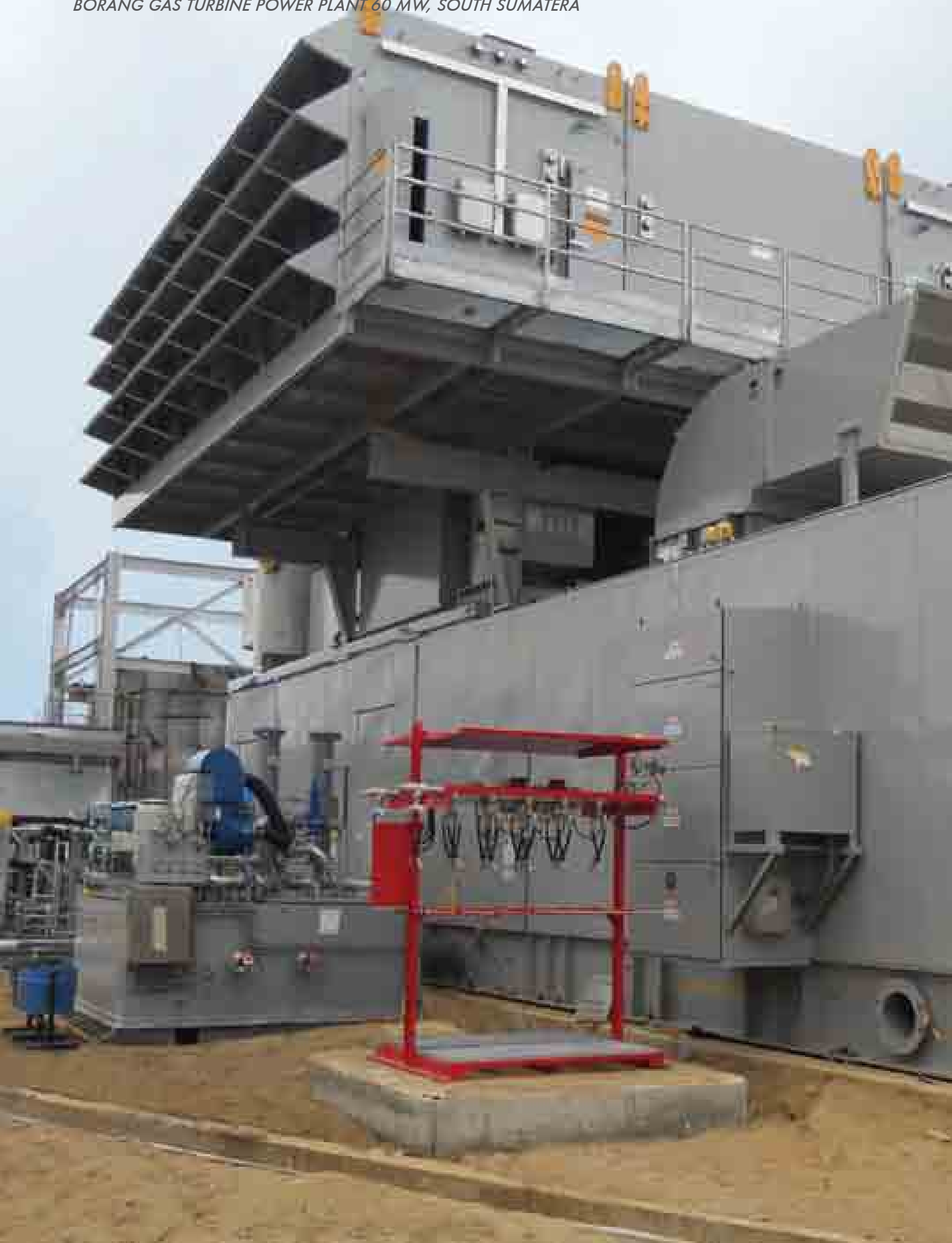
PLTG BORANG 60 MW, SUMATERA SELATAN BORANG GAS TURBINE POWER PLANT 60 MW, SOUTH SUMATERA
